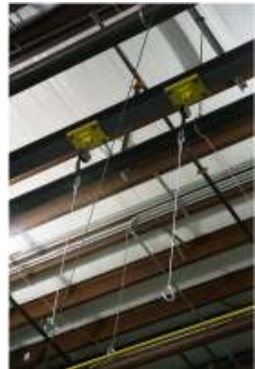
Single Point Anchors attached to a steel truss provide an option for safe maintenance.
