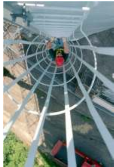
A worker using a vertical lifeline and ladder system to provide maintenance on a tower.
