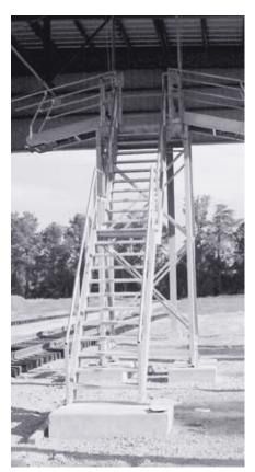
Access platforms, stairs, and gangways are simple, easy-to-use passive fall restraint systems designed to prevent slips and accidents before they happen. Access platform designs can range from single station installations to complex, multi-unit systems. (For loading and unloading applications, the access platform's height must allow sufficient clearance for railcars, tankers, and trucks commonly serviced.)
