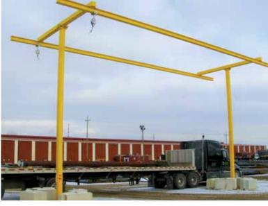
There are two very important design considerations when determining your gallows system. The height of your railcars or trucks establishes your fall clearance, this in turn determines if a rigid or cable system can be used. Also, it is important to know the soil compaction around your tracks so the foundations of the gallows can be designed correctly.
