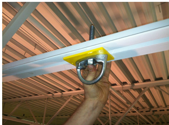
Figure 6 - D-Ring and Bottom Plate Aligned on Truss
