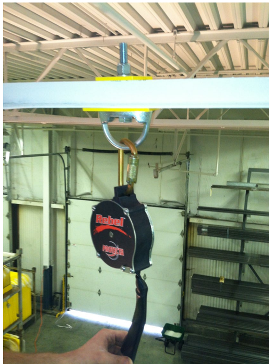
Figure 18 - SRL Attached to FTA via Carabiner
