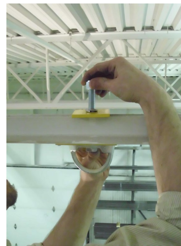
Figure 9 - Lock Nut on Assembly
