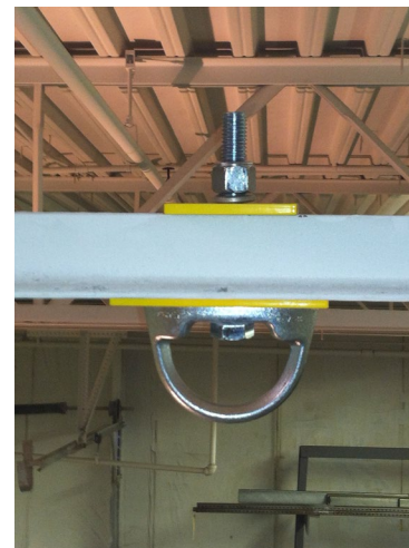
Figure 10 - Proper Assembly of FTA
