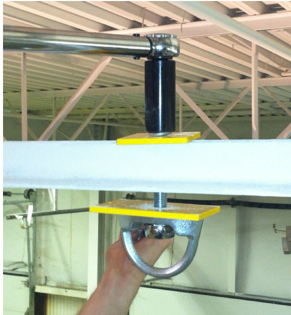
Figure 17 - Torque Lock Nut to 75 ft-lb
