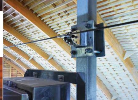
**Above** shows a lifeline system designed specifically for Silo applications.
