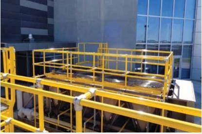
Guardrail systems provide simple and easy-to-use leading edge fall protection for a variety of applications, including rooftops, mezzanines, stairs, access platforms, gangways, and loading docks just to name a few. From freestanding safety railing systems to permanent installations, the safety engineers at DFP can recommend a guardrail solution that will keep your employees safe and your facility in compliance with all OSHA fall protection regulations.
