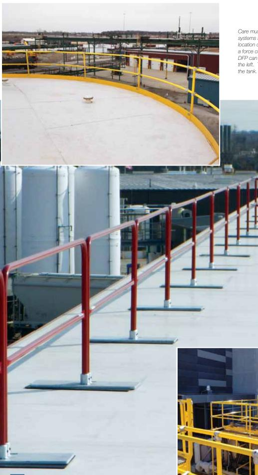
Care must be taken when specifying weighted base guardrail systems to consider loads applied to the deck. Regardless of location or mounting style, the top rail must be rated to withstand a force of at least 200lbs; the mid-rail must be rated at 150lbs. DFP can also make custom guardrail as shown in the photo to the left. The round guardrail was bent to match the radius of the tank
