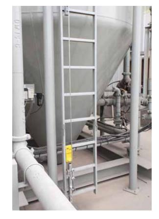
DFP's EZ Series access ladder system meets all of the new OSHA requirements and installs in less time than traditional fixed ladders with welded stand-off brackets. DFP fall protection engineers can help identify your ladder fall hazards, make specific recommendations to increase the safety of your ladder systems, and implement a safety and training program to ensure worker safety and OSHA compliance.
