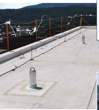
From rooftop tip over posts to specialty vacuum anchors, we offer a wide range of single point anchors (SPA) to meet the needs of different industries and applications. Single point anchors are cost effective and easy to use, making them an ideal fall protection solution for clearly designated work areas in which a wide range of motion is not required.
