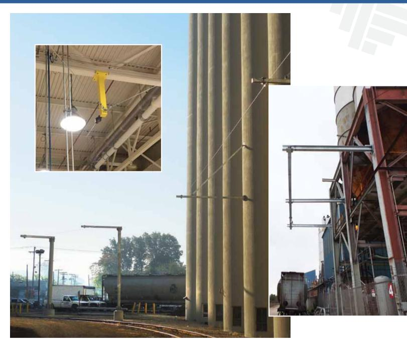
There are two very important design considerations when determining your gallows system. The height of your railcars or trucks establishes your fall clearance, this in turn determines if a rigid or cable system can be used. Also, it is important to know the soil compaction around your tracks so the foundations of the gallows can be designed correctly.
