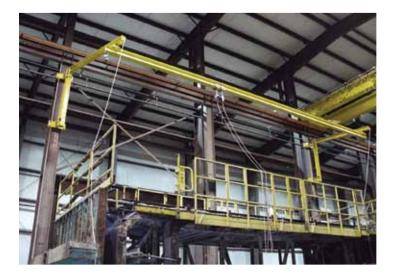
For articulating jib systems, one of the most important design considerations is assessing the total coverage area that will need fall protection to protect workers as they perform routine maintenance and daily job duties. The number of users and the potential need for by-pass capability is also an important factor when developing system specification and design features.
