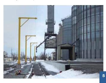
Rigid Rail systems are typically in any application where workers have a very limited fall clearance available. Where Lifeline systems, have deflection in the event of a fall which increases the total fall distance required, rigid rail systems, have little to no deflection giving the worker a safe fall distance in the event of a fall.
