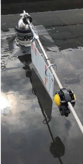
The slope and the construction of your roof are the two factors when determining your rooftop lifeline. No matter the style, all DFP lifelines are a continuous pass-through system that allow workers to travel the entire system length without disconnecting.
