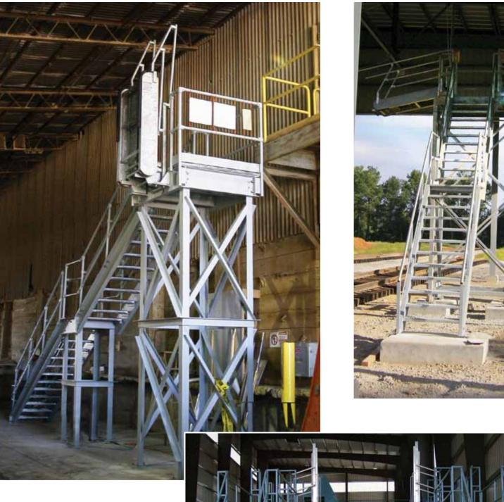
Access platform designs range from single station installations to complex, multi-unit systems. For loading and unloading applications, the access platform's height must allow sufficient clearance for railcars, tankers, and trucks commonly serviced."
