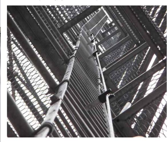
Vertical Lifeline Systems allows movement up and down the entire height of the line, eliminating the need to disconnect and find new tie-off points while ascending or descending from applications like a tower or ladder. By connecting to the vertical lifeline using a deceleration device, users may move as long as tension is slack on the lifeline.
