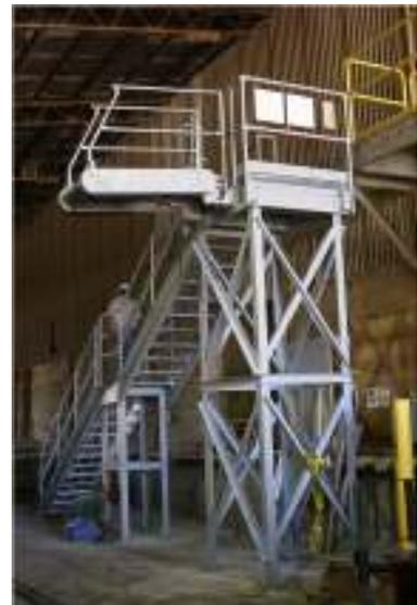
A stairway system with a gangway provides safe access to operations at height.
