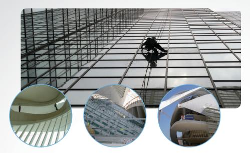
UniRail's strength and functional characteristics make it very suitable for use as an anchorage system for rope access and abseil work tasks where the structure requires inspection and light to medium duty tasks.
