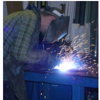
Welders shall have AWS D 1.1 certification when fabricating fall protection systems.
