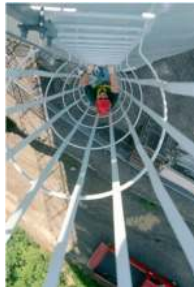
A worker using a vertical lifeline and ladder system to provide maintenance on a tower.
